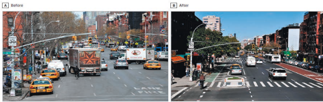
Figure. First Avenue Before and After Bus and Bike Lanes Were Added
